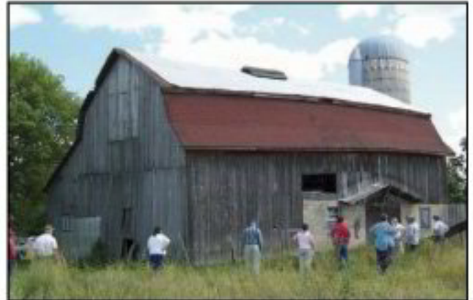
Above: U.P. conferees learn from barnwright Steve Stier, the steps needed to make this Escanaba-area barn good as new.
