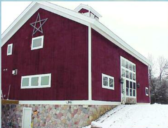
Chris Sayles' Jackson barn house is a work in progress. Learn from Chris at the March conference!
