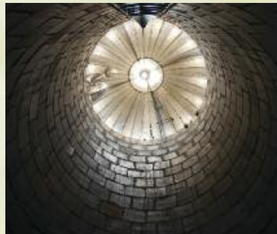
Interior of the silo at the Racich barn.
