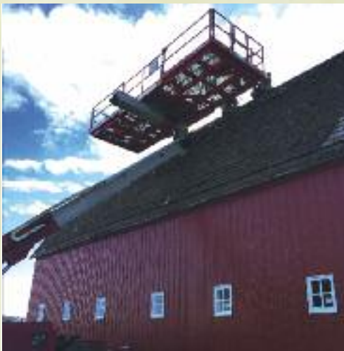
Work proceeds on the Kennedy Barn, rural Saskatchewan, Canada.
