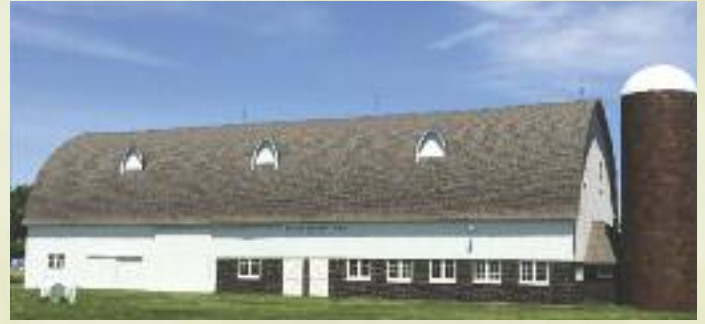
Brandt Barn in Bay City, MI — Most noticeable feature of this 130 ft barn is the gothic style roof covered in asphalt shingles in a color nearly matching the exterior blocks’ dark brown glazed tile.
