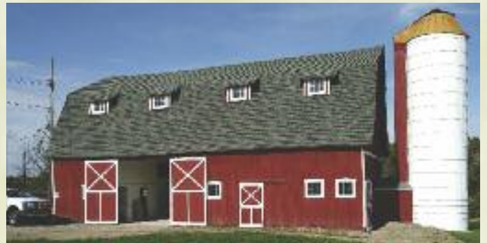
Gierok Barn in Rochester Hills, MI (Oakland County) -- This 30 x 60-foot gambrel-roofed barn at Rochester University has newly installed asphalt shingles matching a historical shingle, a connected silo and tongue and groove wood planking sides
