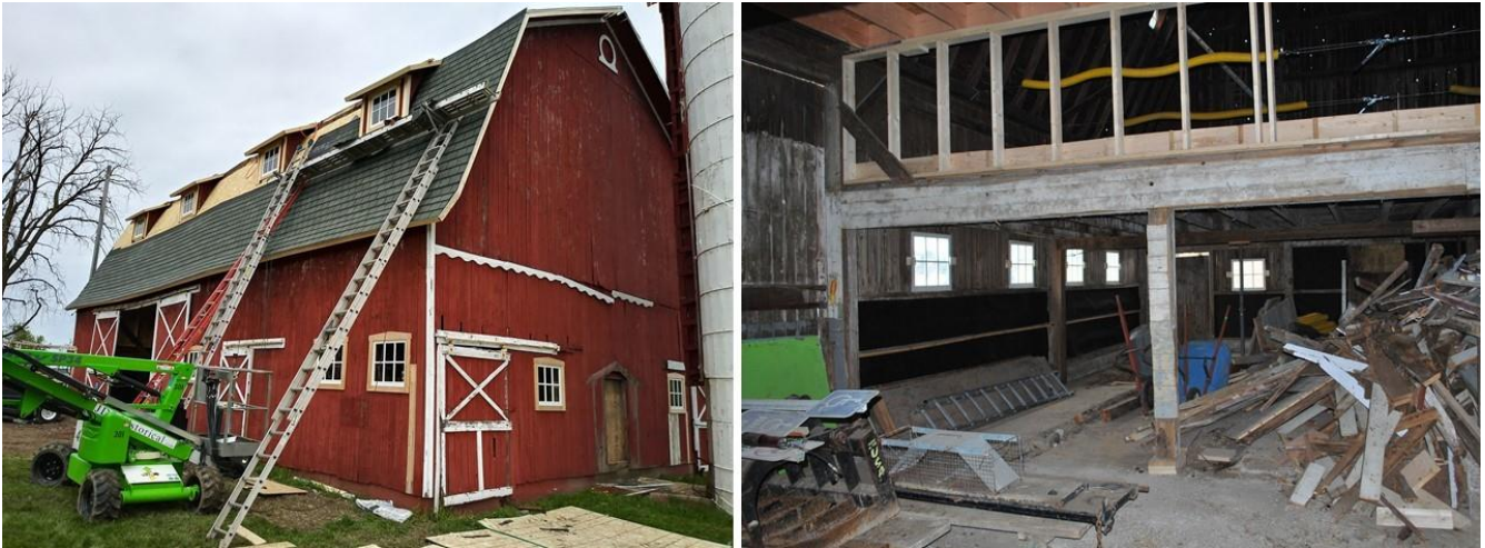
Gierok Barn in Rochester Hills during rehabilitation project
