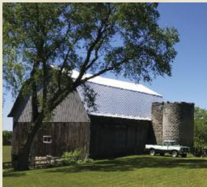
An old barn again made new.
