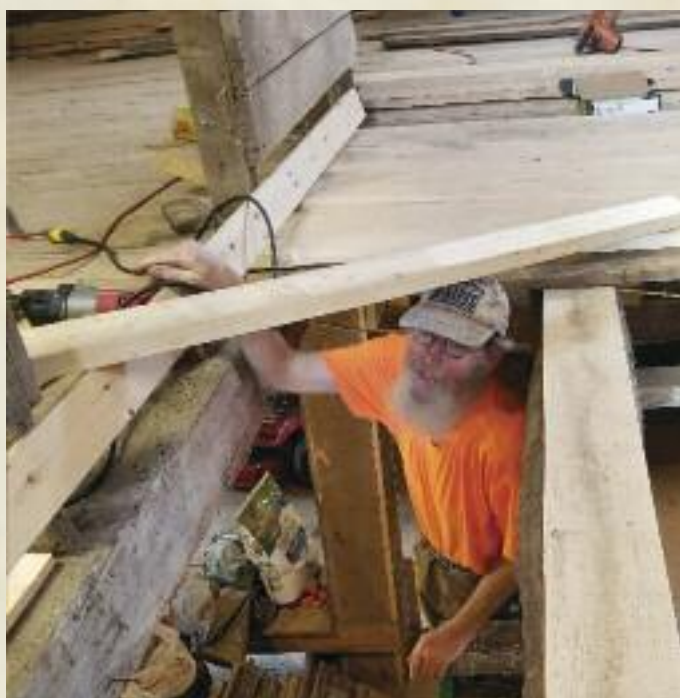
Replacing floor boards
