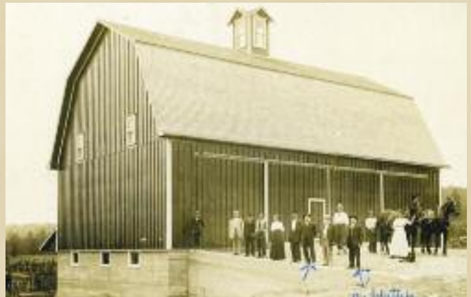
Leelanau County Poor Farm Barn 1911. Builder John Schettek in foreground. The original cupola and shed roof (just visible at lower right in photo) were removed at an unknown date. A generous grant from the Ball Foundation will fund reconstruction of both the cupola and the shed roof on the lower west wall.
