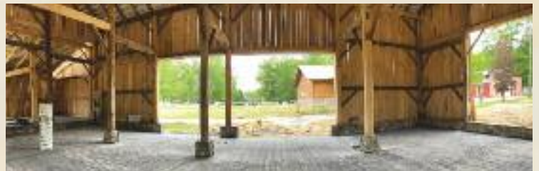
Barn of the Year Award (2022), Interior work on the Griffin Barn (Ogemaw County)
