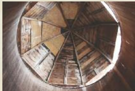
Wood silo roof (interior) at the Gregory Barn
