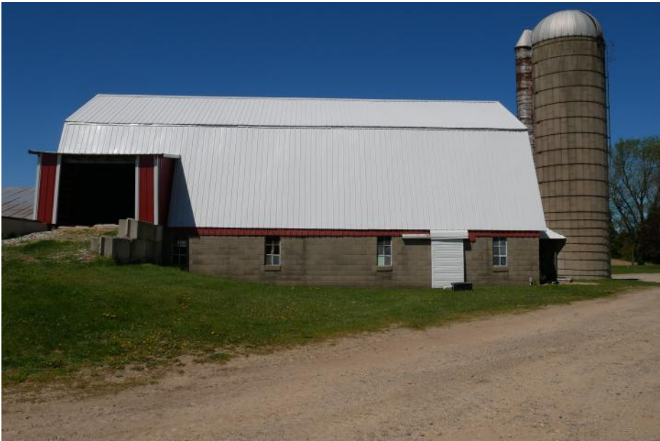
Dhooghe Barn. Concrete block wall at lower level. Plank frame gambrel roof framing. Metal roof.
