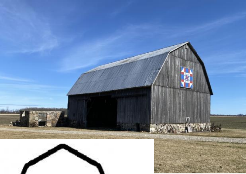
Gambrel roof barn, with stone foundation, plank framing.
