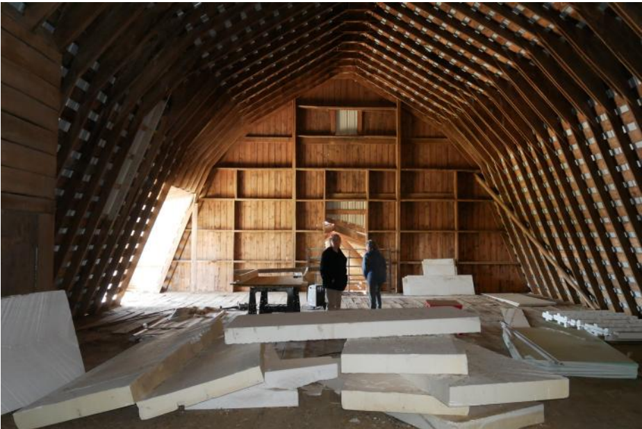
Dhooghe Barn. Concrete block wall at lower level. Plank frame gambrel roof framing. Metal roof.
