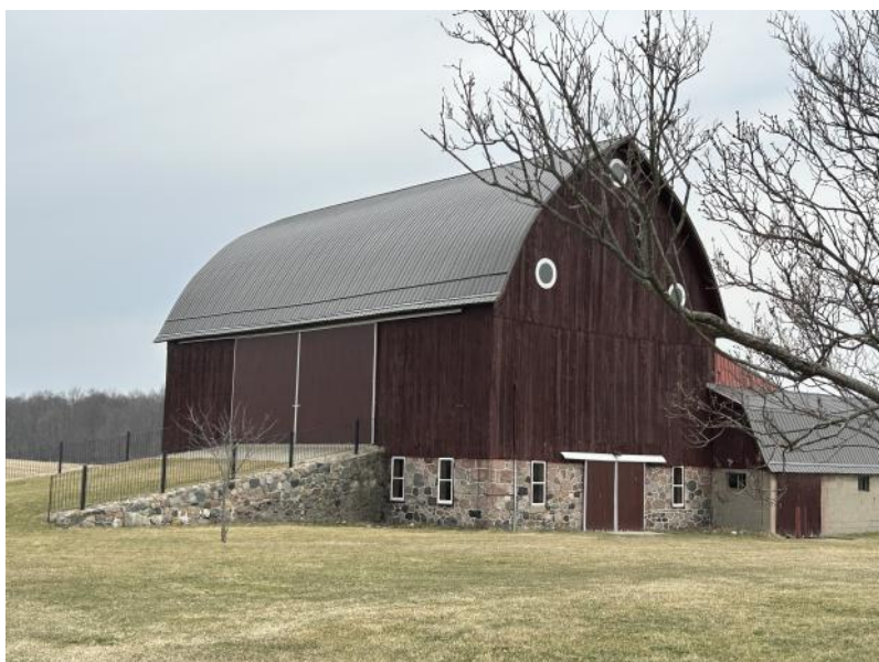
Raised ramp, arched roof barn with stone foundation.
