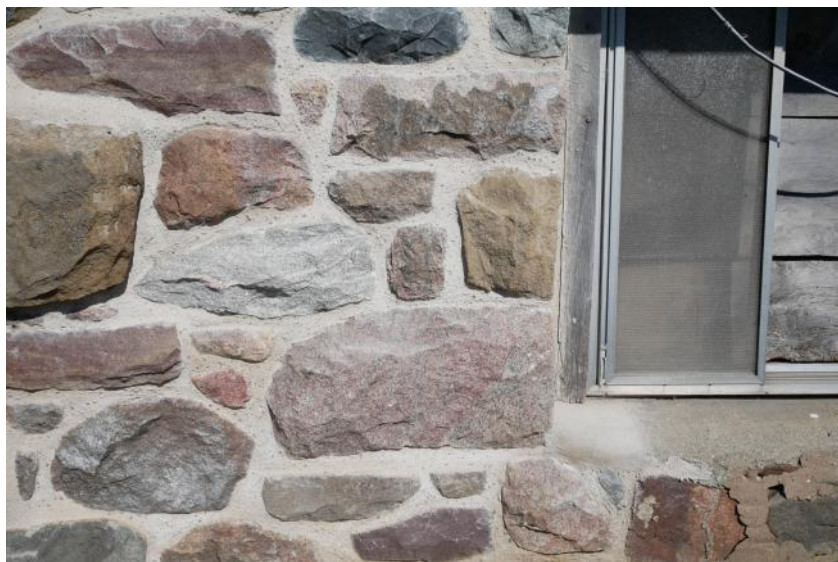
Beautiful stone repair by MBPN contractor member; Schmitt & Sons Stonework.
